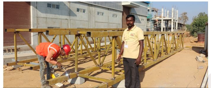
ELECTRICAL & METAL FABRICATION WORKS
