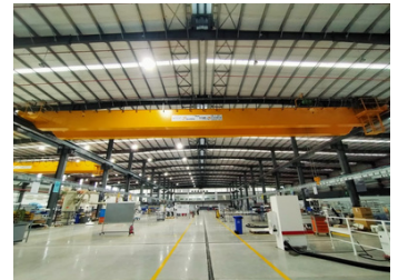
Homag Shop Floor Highbay Lighting
