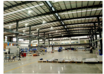
Homag Shop Floor Highbay Lighting
