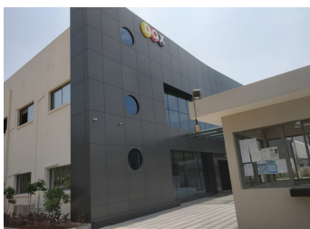
DCX CCTV Installation
