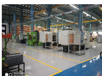
Trelleborg BBT & High Bay Lighting
